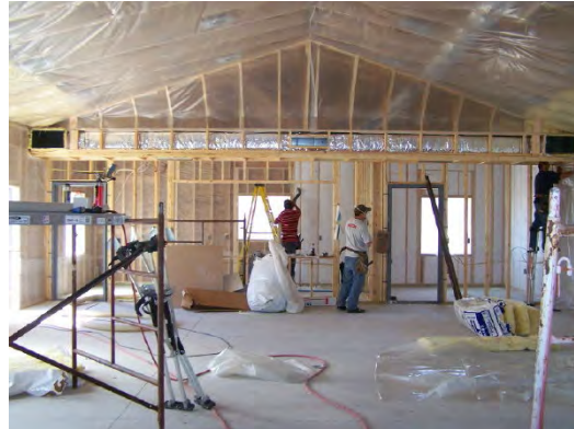
Installation of insulation in Canterbury Room.
